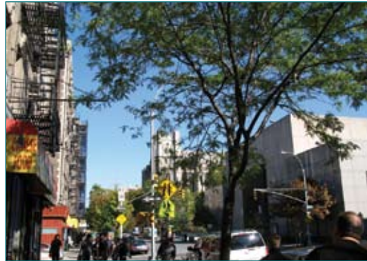
Manhattan's West Side hosts a major stone edifice—and the substation designed to harmonize with it.
