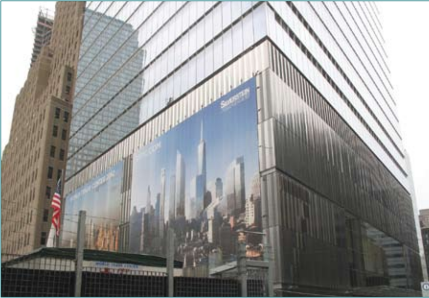
The office floors of 7 World Trade Center sit atop Con Edison's Trade Center Substation, a major electrical distribution point for lower Manhattan. Changing zoning restrictions would enable New York to install more substations like this.
