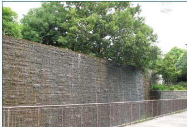
"Nagoya people love waterfalls," said a Chubu Electric engineer as he pointed out the cooling and noise-camouflaging feature on the side of the Meijo Substation ventilation building that faces the castle (bottom). Another waterfall hides the subpark area-level (154kV/33kV) substation that preexisted the magnificent transmission-level (275kV/154kV) Meijo Substation across the street.
