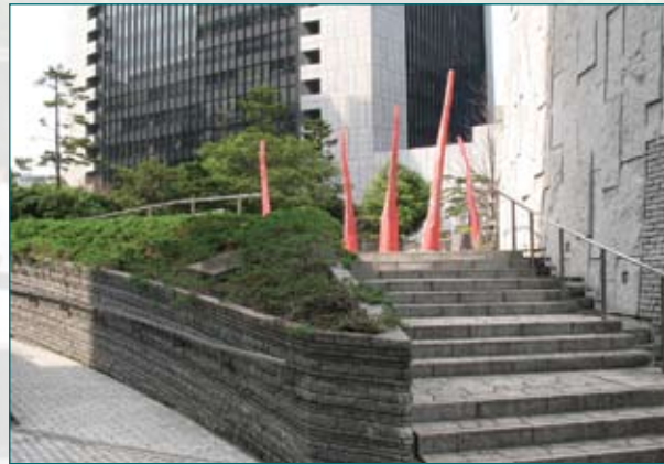
The transmission-level (275kV/66kV) equipment at Higashi-Uchisaiwai-cho Substation is located mainly under TEPCO's own building (top) and forecourt in congested central Tokyo. Other facilities, including space to install an area-level substation in the future, lie beneath the adjacent public concert plaza (bottom).
