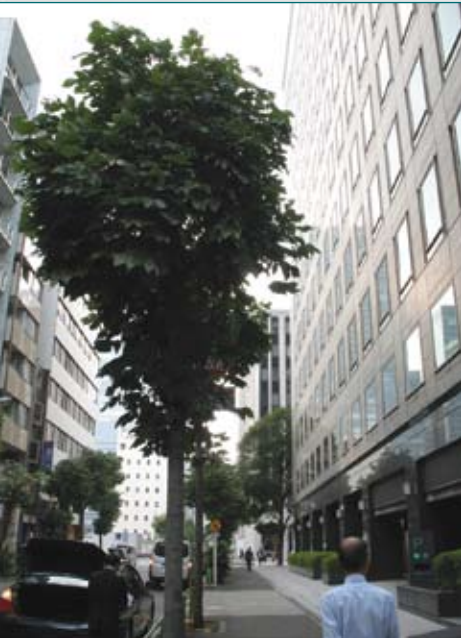
Minami-Saya-cho Substation lies beneath the office tower at right, near Tokyo's Ginza. On line since 1997, the substation houses two 66kV/22kV transformers for distribution to major commercial customers, as well as two 66kV/6.6kV transformers for local distribution.
