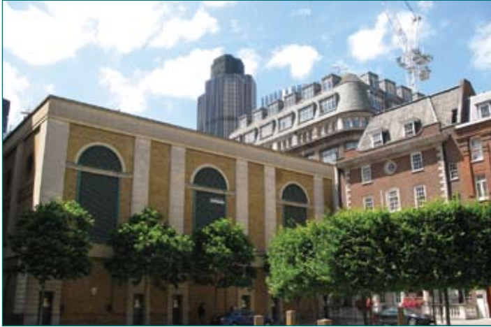
The rear of this substation has provided one of the walls of London's Devonshire Square since the late 1970s. The substation's front yard is Jubilee Gardens, a landscaped seating area that camouflages the switchgear vents.
