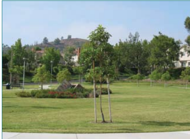
Anaheim Public Utilities took advantage of sloping topography to build the 69kV/12kV Park Substation into the side of this hill—topping it off with a manicured public lawn.
