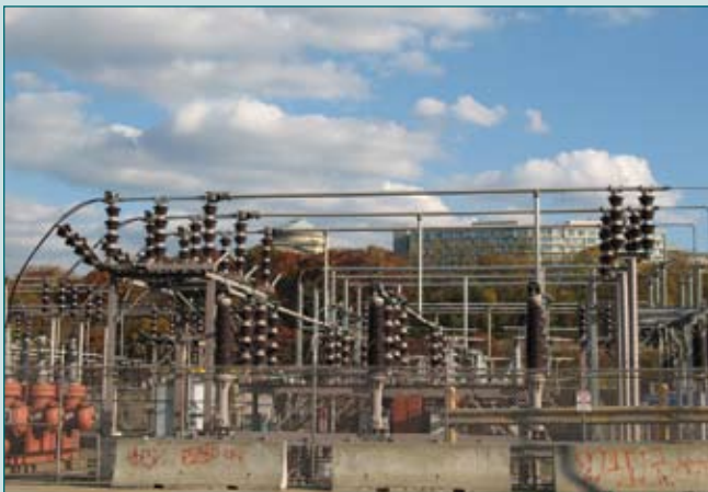
Con Edison's East Yard blocks access to the Harlem River...
