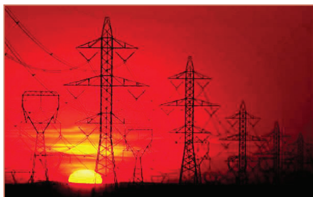
figure 2. Transmission lines gallop across the landscape.
