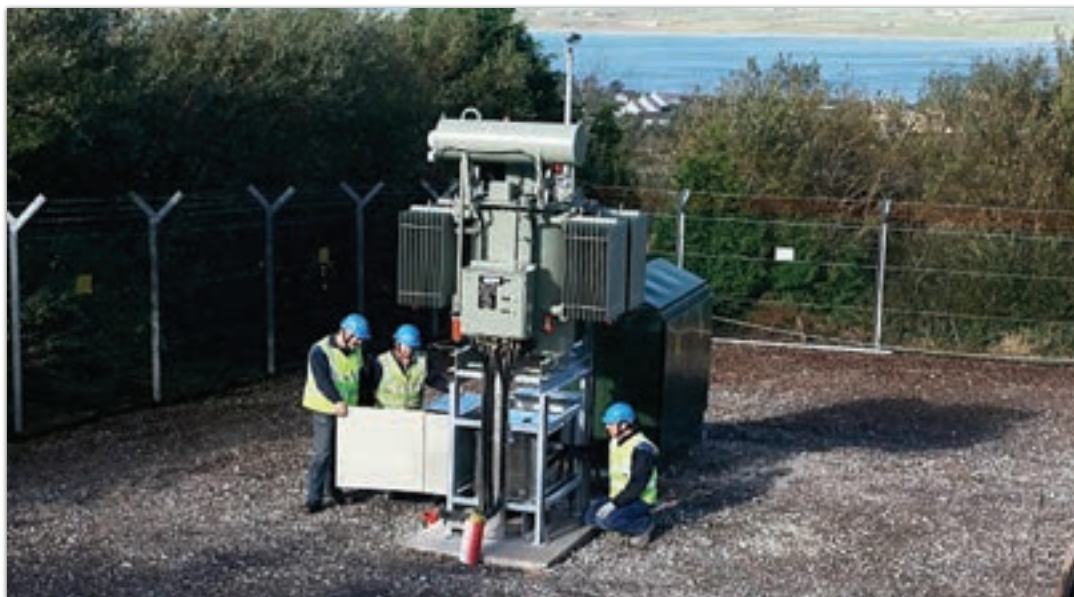
Arc Suppression System at Gurranbane Substation
