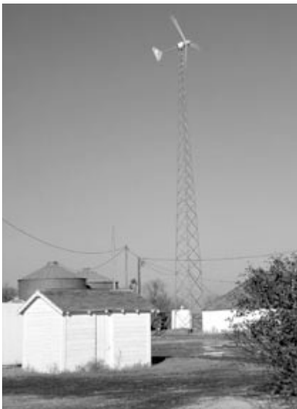
Warren Gretz, NREL/PTW09634
