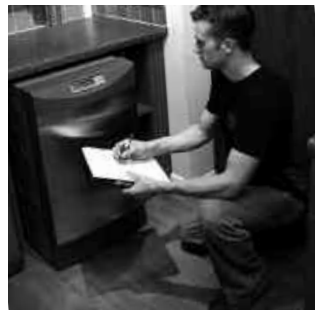
A micro-CHP unit, replacing a floor-standing central heating boiler © Powergen
