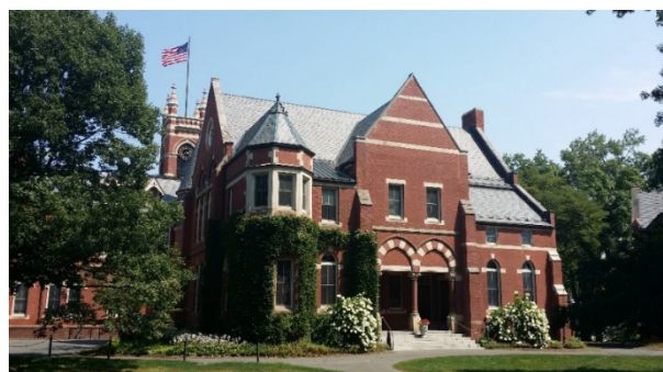
Left: College Hall. Arches in red sandstone and Indiana limestone. Windows trimmed with Indiana limestone. Built by Peabody & Stearns, 1875.
