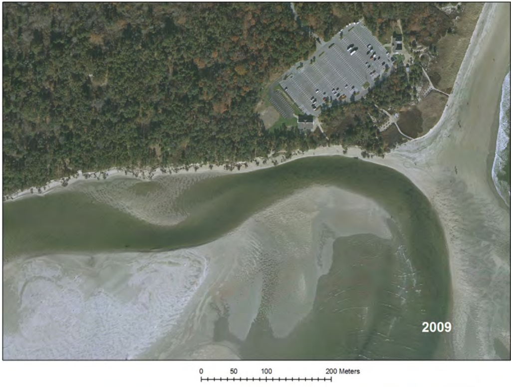
Figure 2: Aerial photo from 2009 showing major erosional event. North is up.
