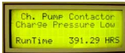
Figure 5-7: Example of Pump Fault Condition Appearing on Keypad Display
