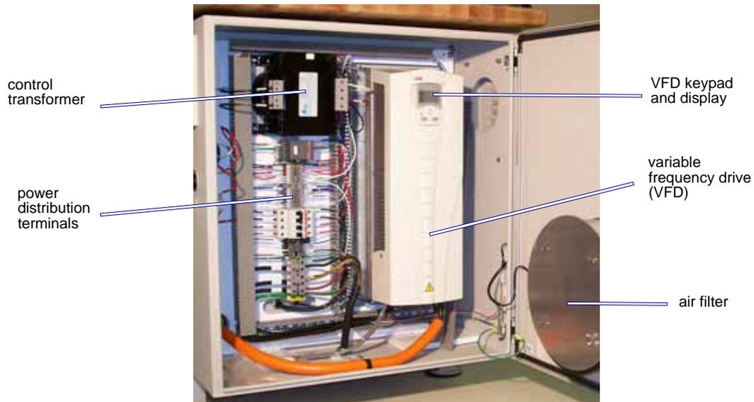
Figure 3-6: Pump Internal Components on Right Side
