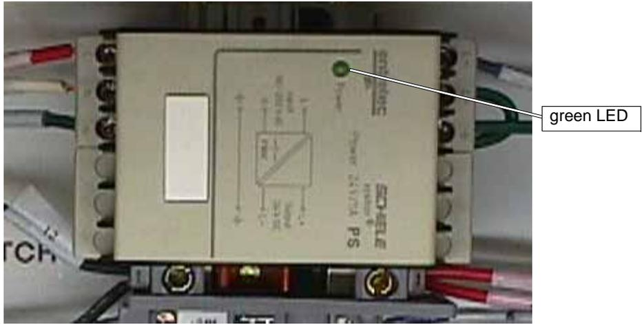
Figure 5-9: 24 VDC Power Supply
