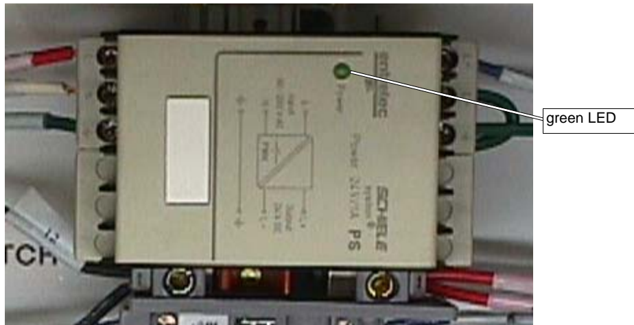
Figure 8-7: 24 VDC Power Supply
