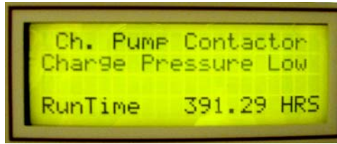
Figure 8-1: Example of Pump Fault Condition Appearing on Keypad Display
